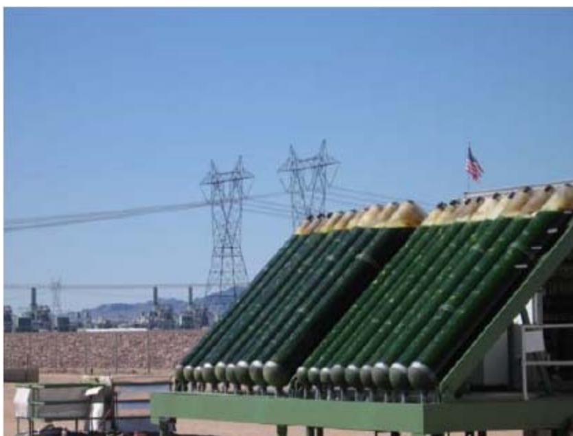
Figure 9-2: Algae bioreactors at an Arizona Public Service power plant (Source: APS: [3])
